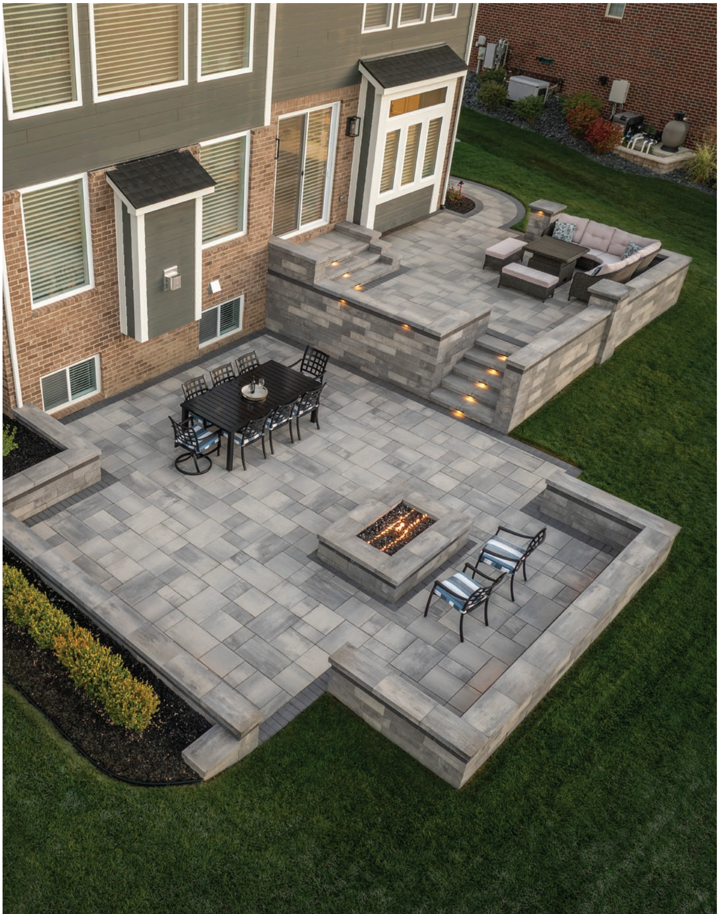
Slabs/Pavers: Nueva® 60mm, Marble Grey with Classic Paver, Onyx border Walls/Fire pit: Nueva® 150 Wall, Marble Grey with Nueva® 75 Wall, Onyx accent Coping/Step Treads: Nueva® Coping, Marble Grey
